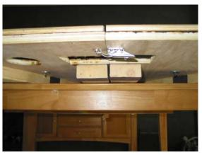
While the little octagon is in place, mark off the edge of the little octagon using a pencil. Remove the little octagon and place some blue painters tape inside the pencil line. You have masked off the race track area and it's time to apply the clear polyurethane.
